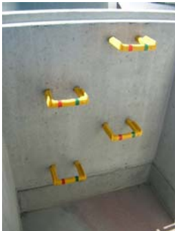
Step irons at 300 mm spacings
