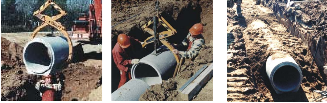
Figure 7: Installation of a drainage pipe
