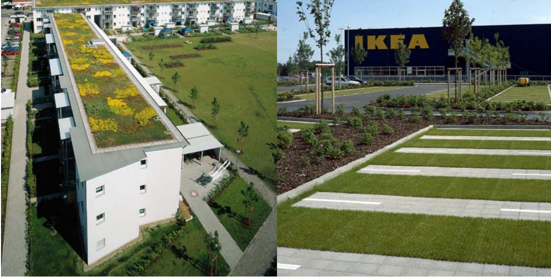
Figure 8: Left: Eco buildings (low energy consuming, greywater reuse) with green roofs, permeable car parks, infiltration pipes for the roof runoff, Right: Permeable car park in front of a furniture store
