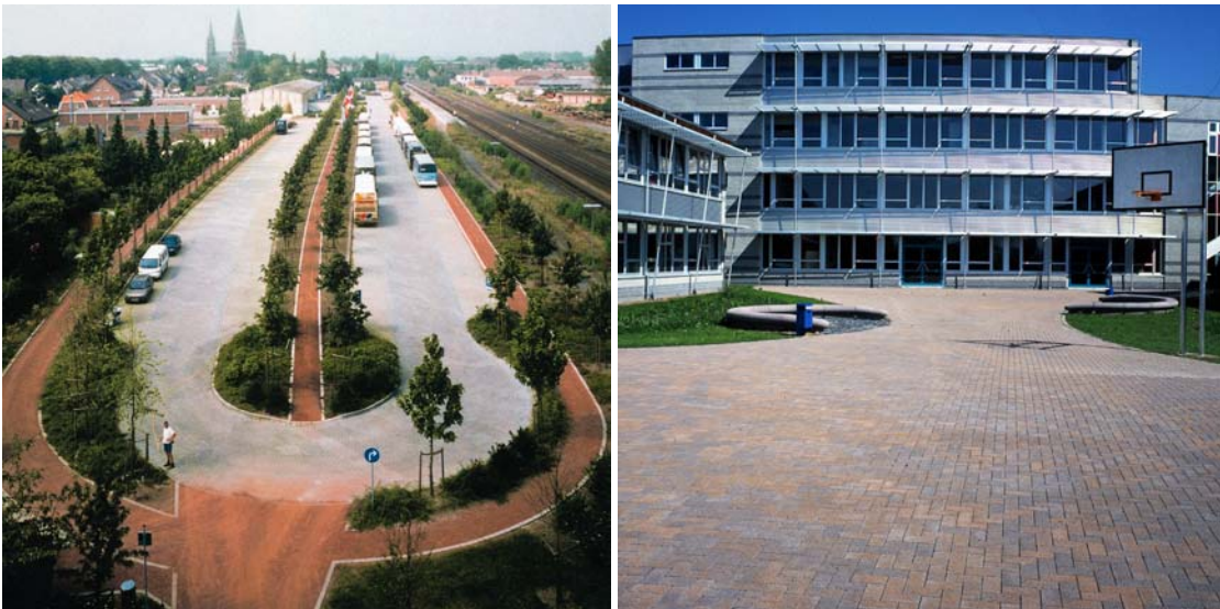
Figure 9: Left: Large bus park and Right: school yard with permeable pavements
