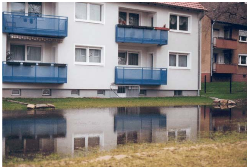
Figure 6: Example of swale with wrong design parameters
