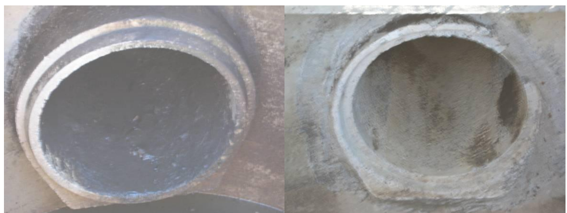
Figure 5. Porous Concrete Pipe – Before (Left) and After (Right) Cleaning
