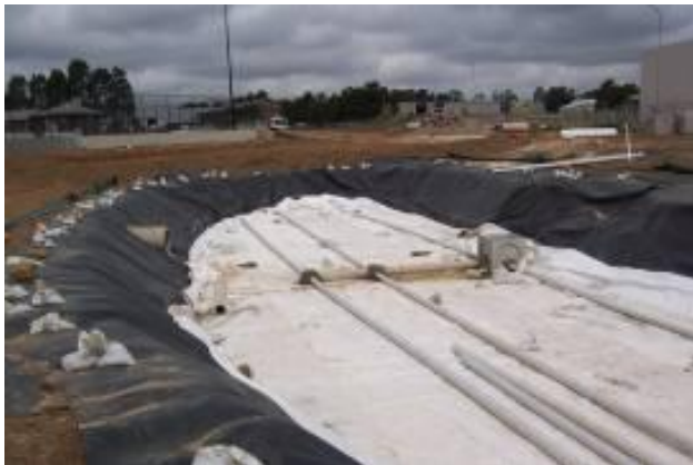
Figures 8 & 9: Ashgrove's Basin A under construction showing liner, HydroCon pipes in position
