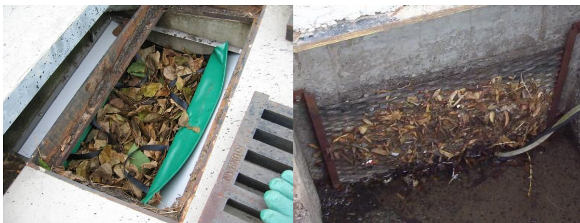
Figure 6. Leaf Accumulation in Pre-Filtering Devices (Left: Asquith; Right: Kiama)
