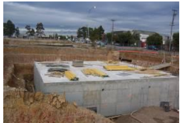
Figure 11: Ashgrove's 800kL treated stormwater storage tank under construction
