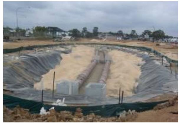
Figures 8 & 9: Ashgrove's Basin A under construction showing liner, HydroCon pipes in position
