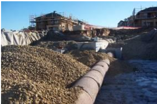
Figure 10: Ashgrove's Basin A under construction showing gravel matrix
