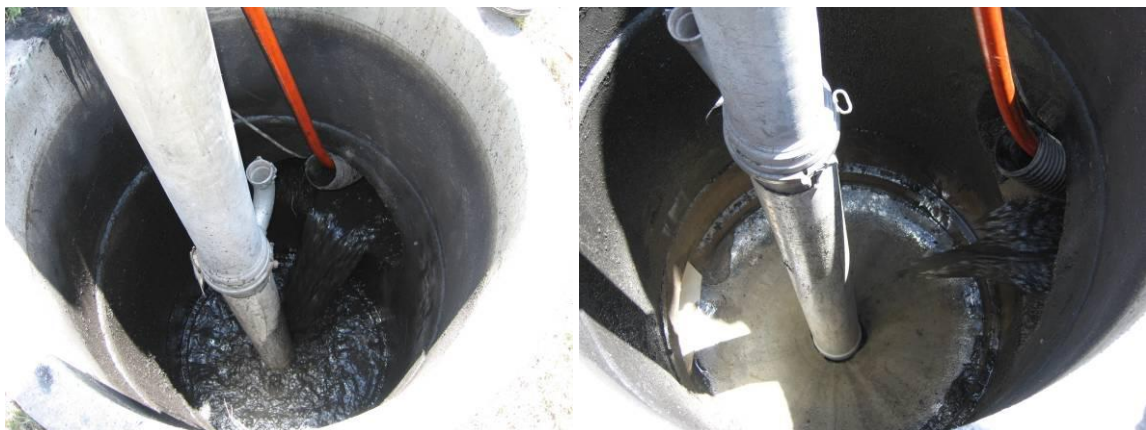
Figure 4. Cleaning of the Heatherbrae System
