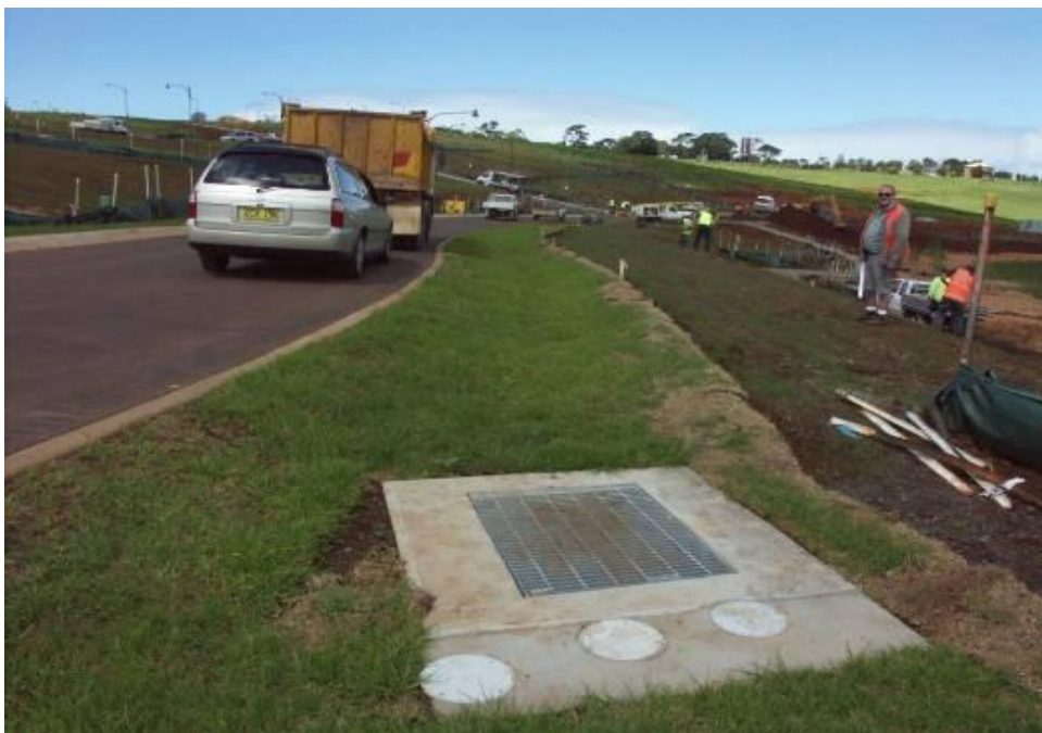
Figure 12: Ashgrove subdivision under construction showing the stormwater system comprising Exfiltration STSs in series
