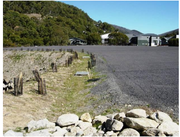
Figures 19 & 20: Thredbo WSUD car park with linear Exfiltration STSs on the perimeter
