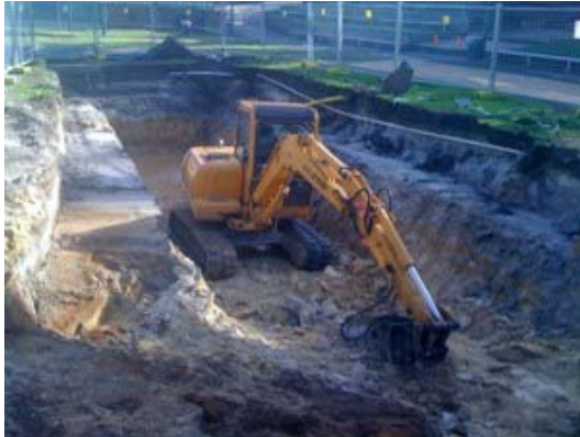
Figure 1 Preparing trench for underground water storage
