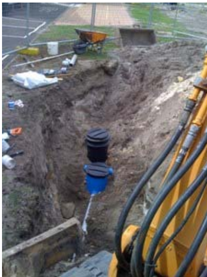
Figure 3 Installing HF400 unit and silt trap
