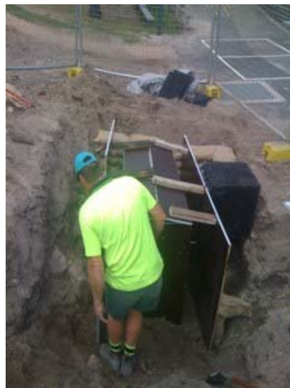
Figure 6 Forming up concrete pit for HF400 unit
