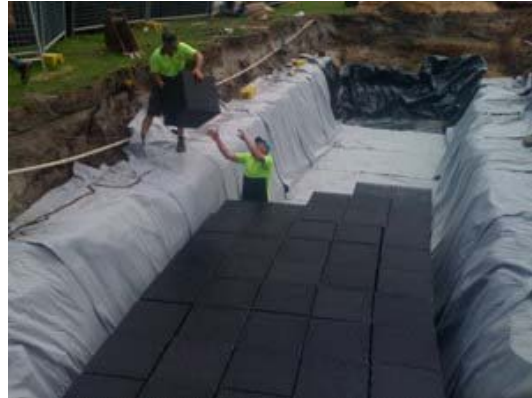
Figure 2 Installing underground VersiTank. Storage tank located approx 10 m from HF400 unit
